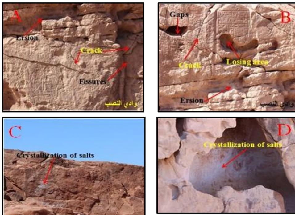
**Fig. 3:** Represents deterioration phenomena of the rock art in Wadi Nasib in Sinai A: erosion and cracks B: missing parts, cracking and gaps, C: crystallization of salts D: crystallization of salts into the gaps.
