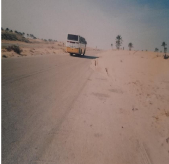
Fig. 25: Sand dune encroachment on the international high way before 2005
