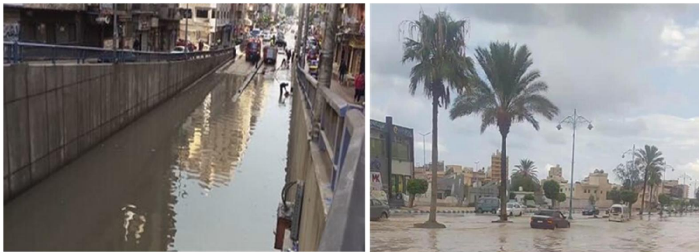
Fig. 7: Photos of flood in Marsa Matruh city at Oct. 2023
