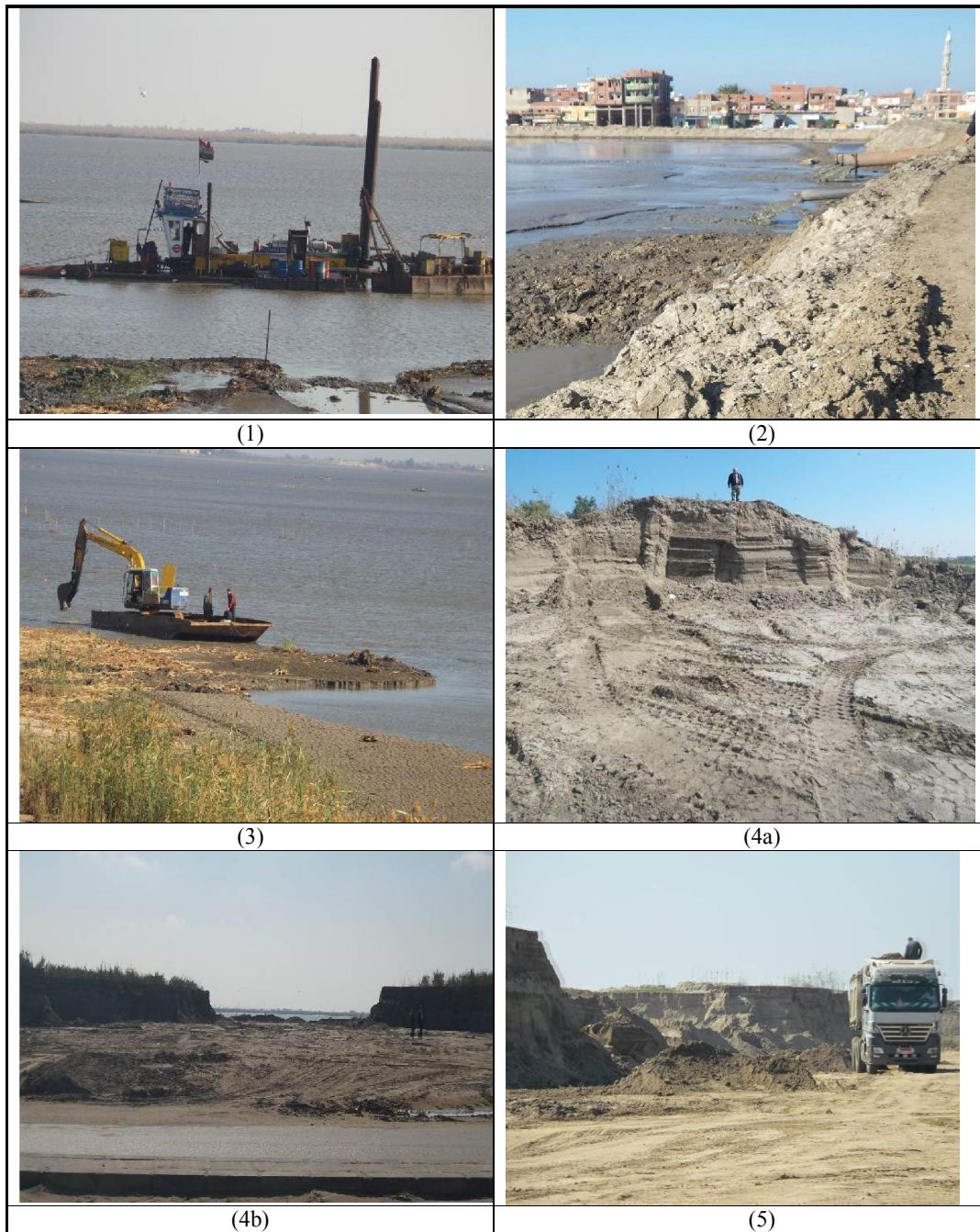
Fig. 2: Showing stages of deepening and cleaning of El Burullus lake.
